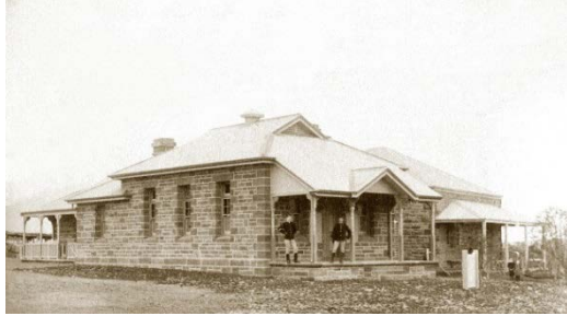
Figure 1 Milparinka courthouse constructed in 1896
